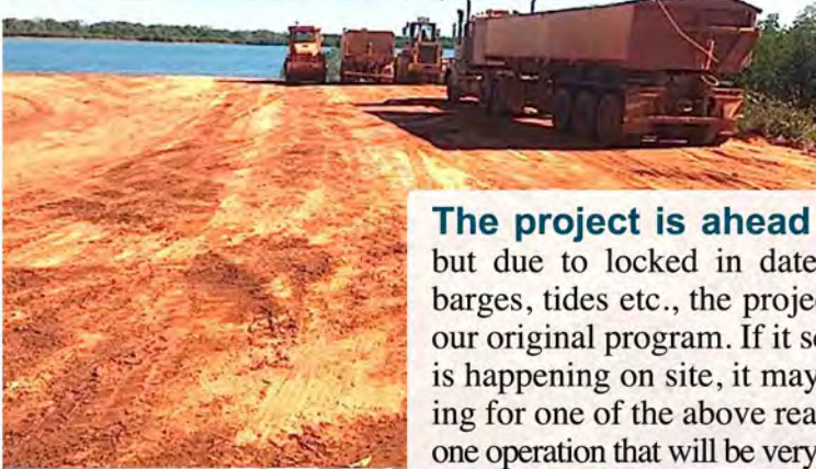
Paru area has been widened and built up.
