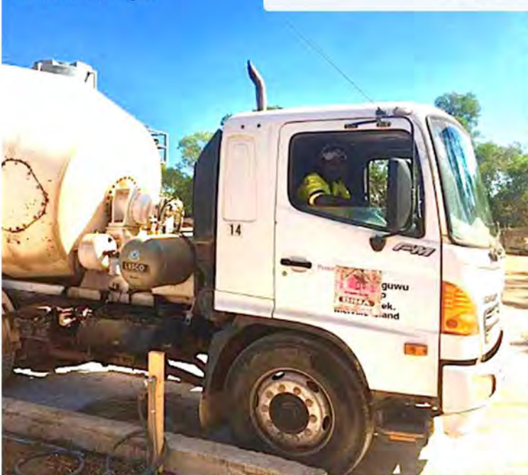
BIHA delivering concrete to the Visitor Centre Project
